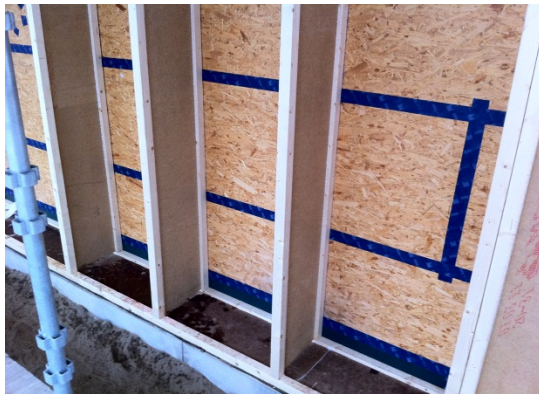
Figure 2: I-joists in the main insulation layer
