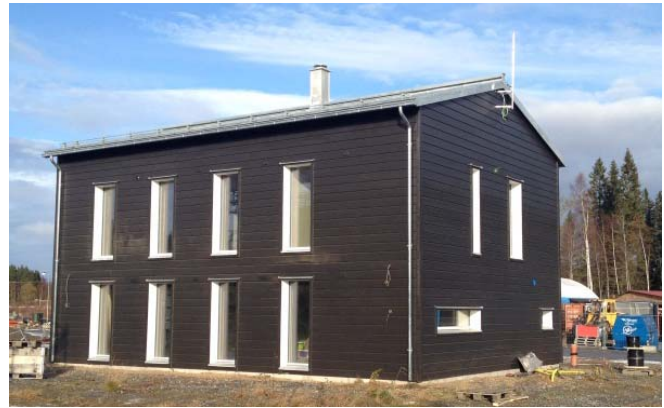
Partway through construction (without shading system) (photo: Greindl)
